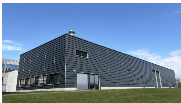
(a) Test hall of the E.ON Energy Research Center in Aachen, Germany
